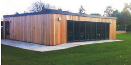
CEDAR-CLAD MODULAR BUILDING
